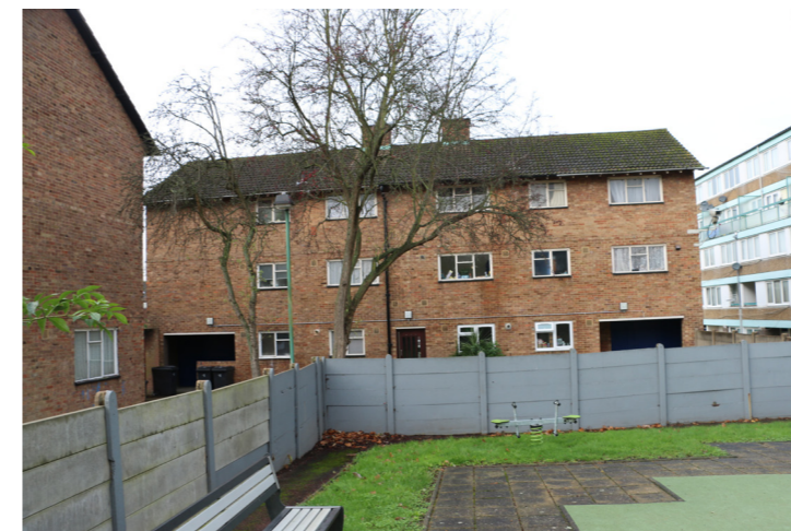
Figure 31 Low rise blocks off Vincent Road
